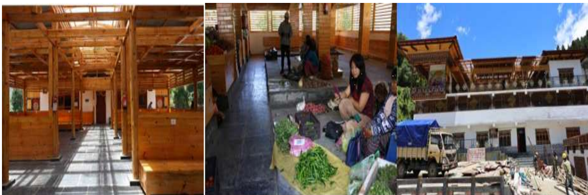
Figure 12: Snapshot of upgraded market facility at Trongsa
